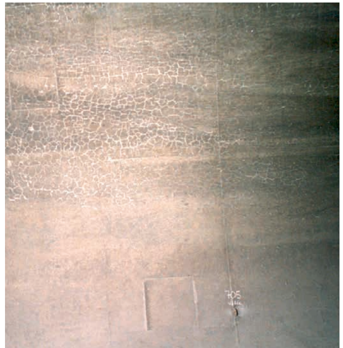
Figure 2 : faïençage dense
